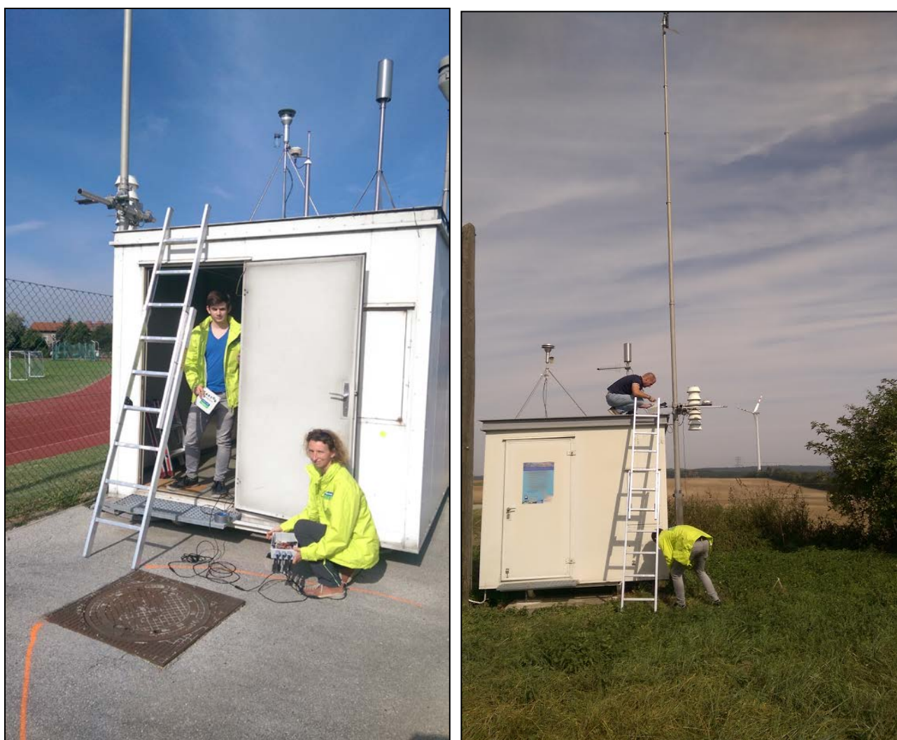
Figure 6: Captor nodes installation in Official Monitoring station in Austria
